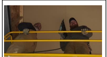
Steve and Stephen West doing ceiling work at Regent Life Church.
