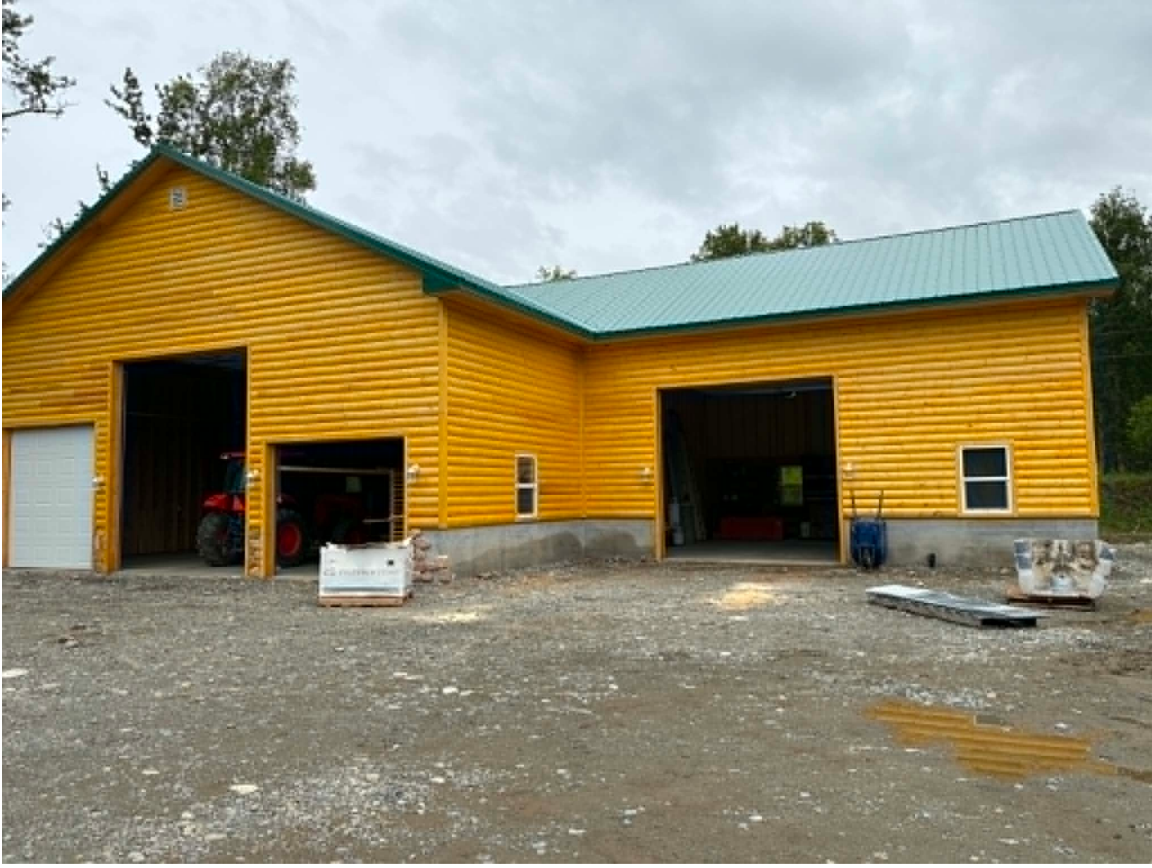
Siding finished on maintenance garage.
